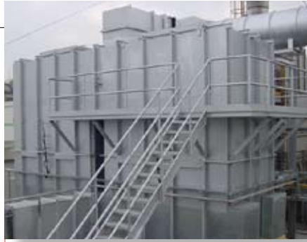
Enterprise Narrow unit 15,000 SCFM EIIN-150 Rooftop installation
