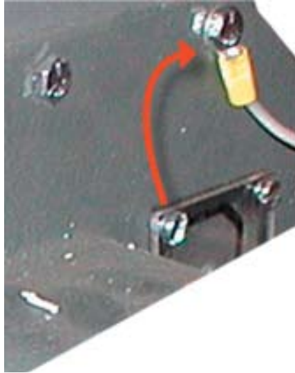
Figure 5. Relocate the flamerod ground wire from the site port screw to the burner casting bolts
